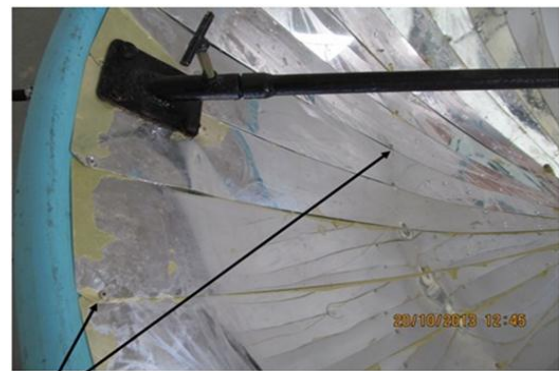
Rivets joining reflector strips to FRP dish
