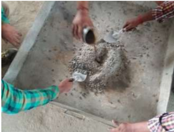
Fig. 2: Mixing of chemicals
