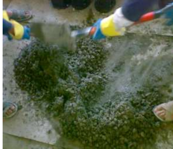
Fig. 2: Mixing of ingredients for making concrete.
