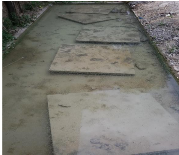
Fig. 4: curing of slab
