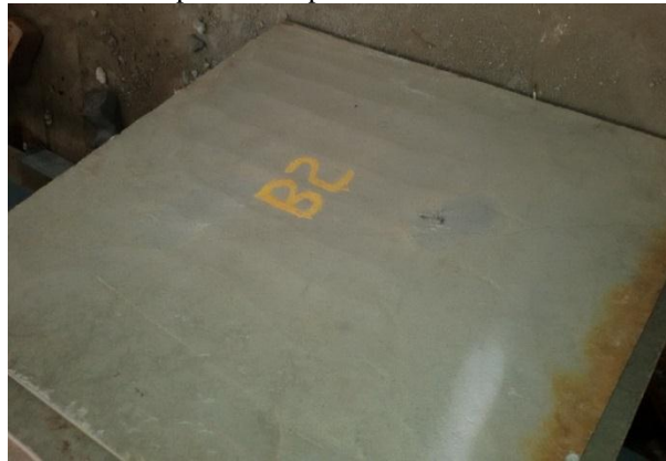
Fig. 7: crack pattern on the surface
