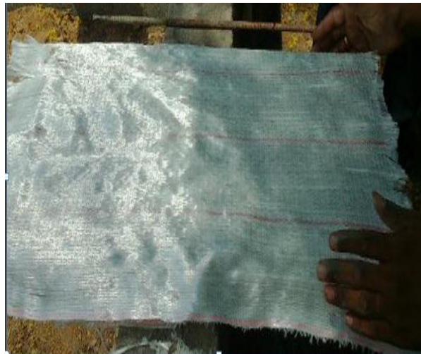
Fig. 5: Application of GFRP layer
