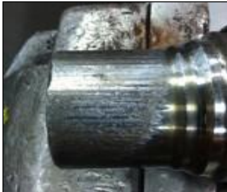
Fig. 3: Universal Joint Spalling (3)
