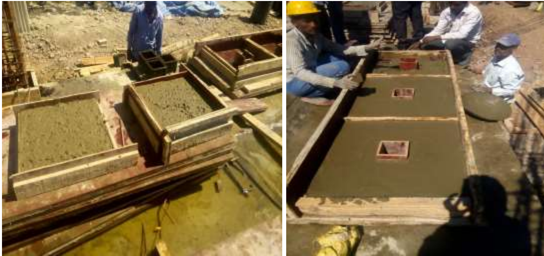
Fig. 2: Slab panels casted on site
