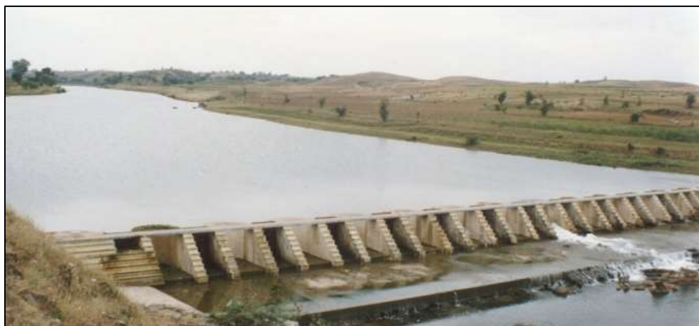
Fig. 1: Bambela Check Dam
