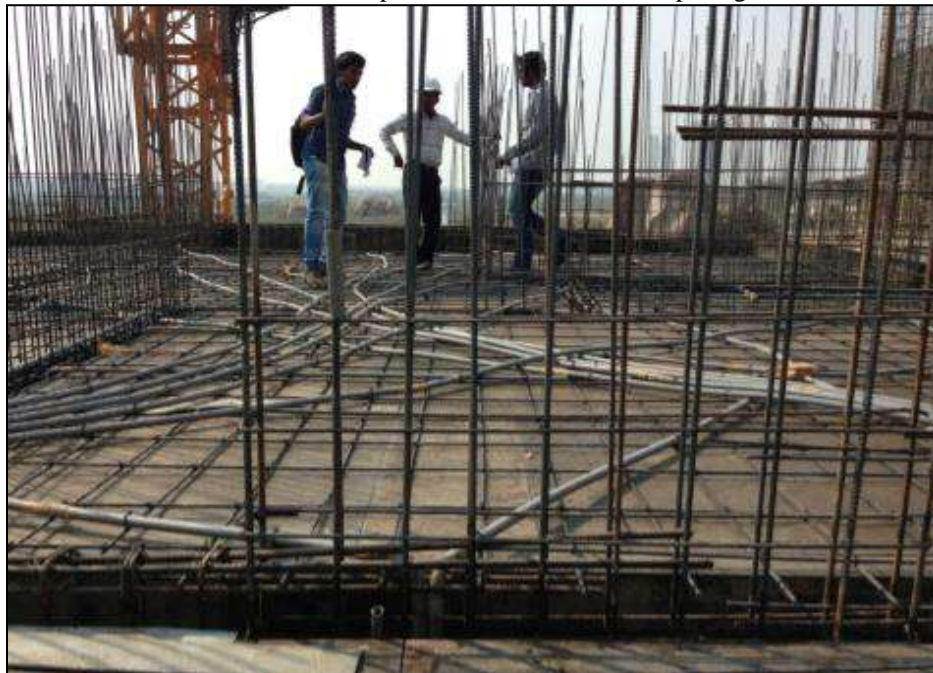
Fig. 7: Vertical Reinforcement of shear wall
