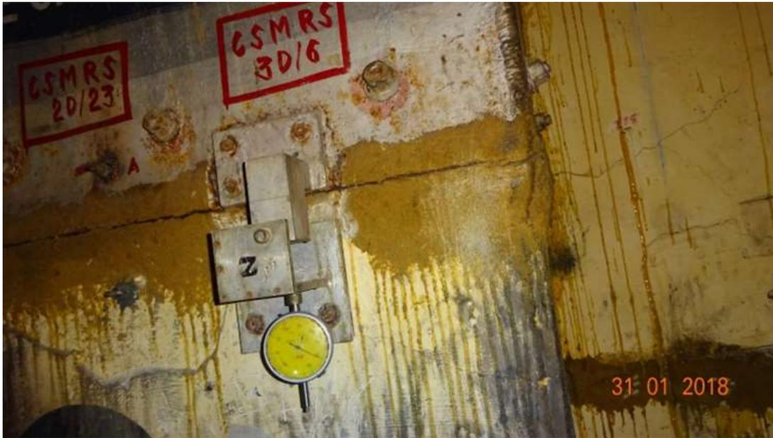
Fig. 2: Location of both instruments on column no.6 at EL 622.00 ft.
